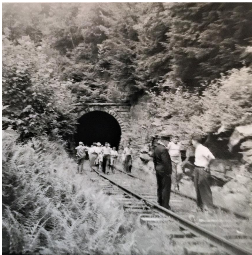
East End of Paddy Mountain Tunnel
