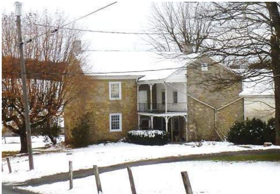
Figure 30 Back of the Clingan House showing stone kitchen with two story porch. The rear of the Thomas IV Barber house has been extensively altered and added on to, but it probably had a covered porch at the ground floor, and possibly a two-story porch similar to this one on its rear wing.
