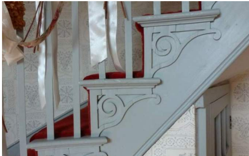
Figure 32 Step bracket trim of circular stair in the Thomas IV Barber house, based on builder's manual.
