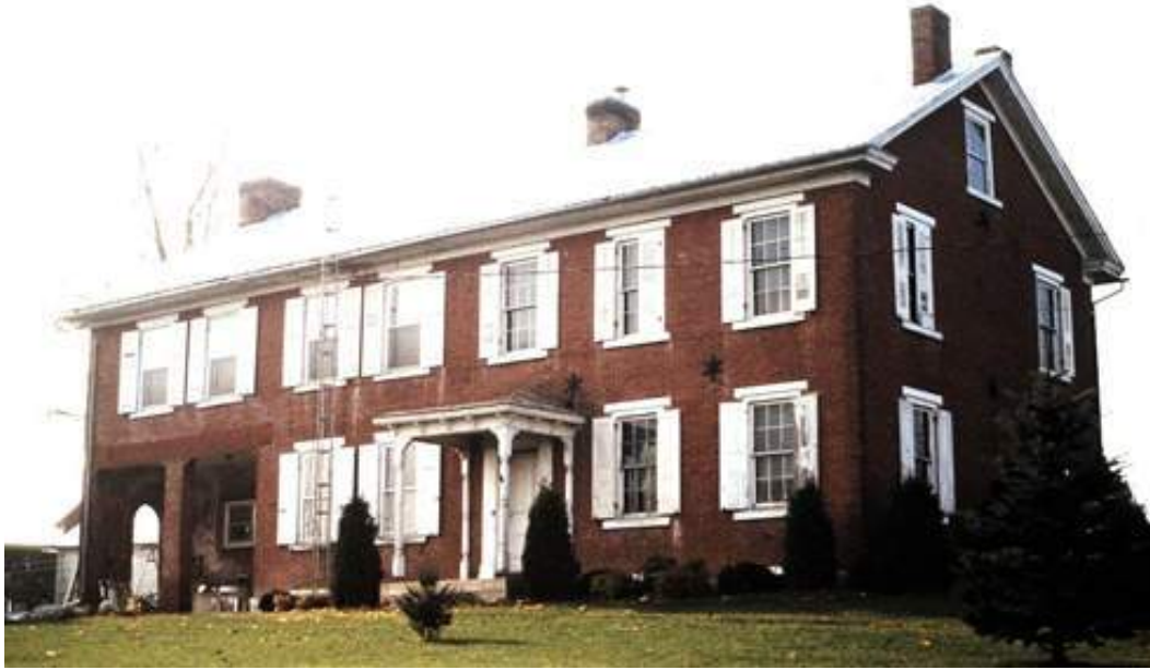
Figure 18 Dr. Robert Van Valzah house, Buffalo Crossroads, in 1983 photo. An original side-hall brick house (on right) expanded to the full five-bay Georgian form, plus an additional two bays.
