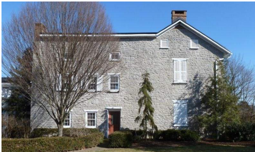
Figure 23 The kitchen wing extending in back of the Thomas IV Barber house has a shed roof rather than the typical gable roof, providing a third floor of back bedrooms tucked under the sloping eaves. Closed false shutters that give the impression of windows below the chimney are a curious original feature of the house.
