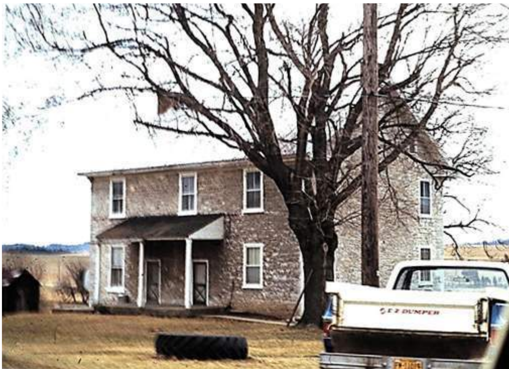
Figure 14 Rear of the Samuel IV Barber house in 1985 photo showing less formal fenestration with low doorways. Large window with low sill on the left illuminates the kitchen.
