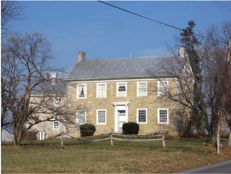
Figure 29 The 1795 Clingan House in Kelly Township, a stone central hall I-house, viewed from south
